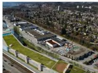
NORTH SHORE WASTE WATER TREATMENT PLANT
