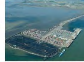
PORT OF VANCOUVER TERMINAL EXPANSION
